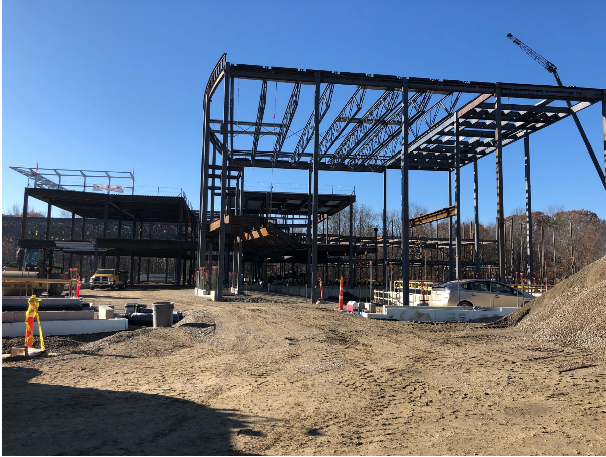
Erected Steel at Auditorium to Roof
