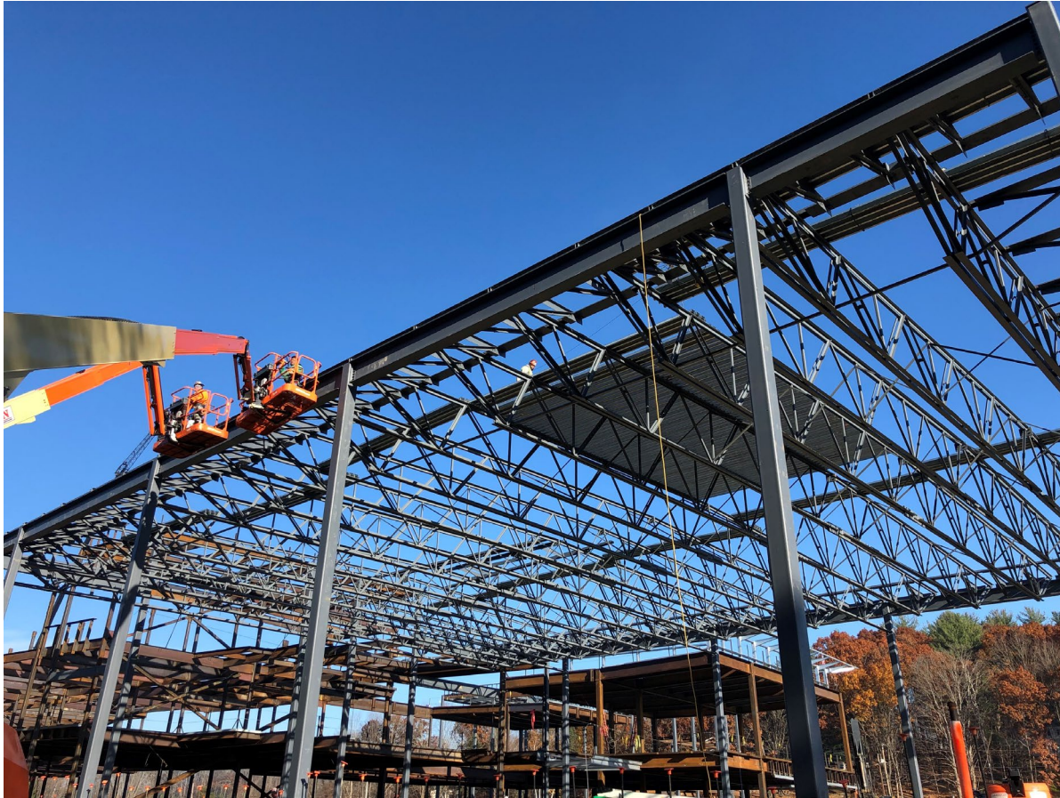
Installing Steel and Decking at Gym Roof
