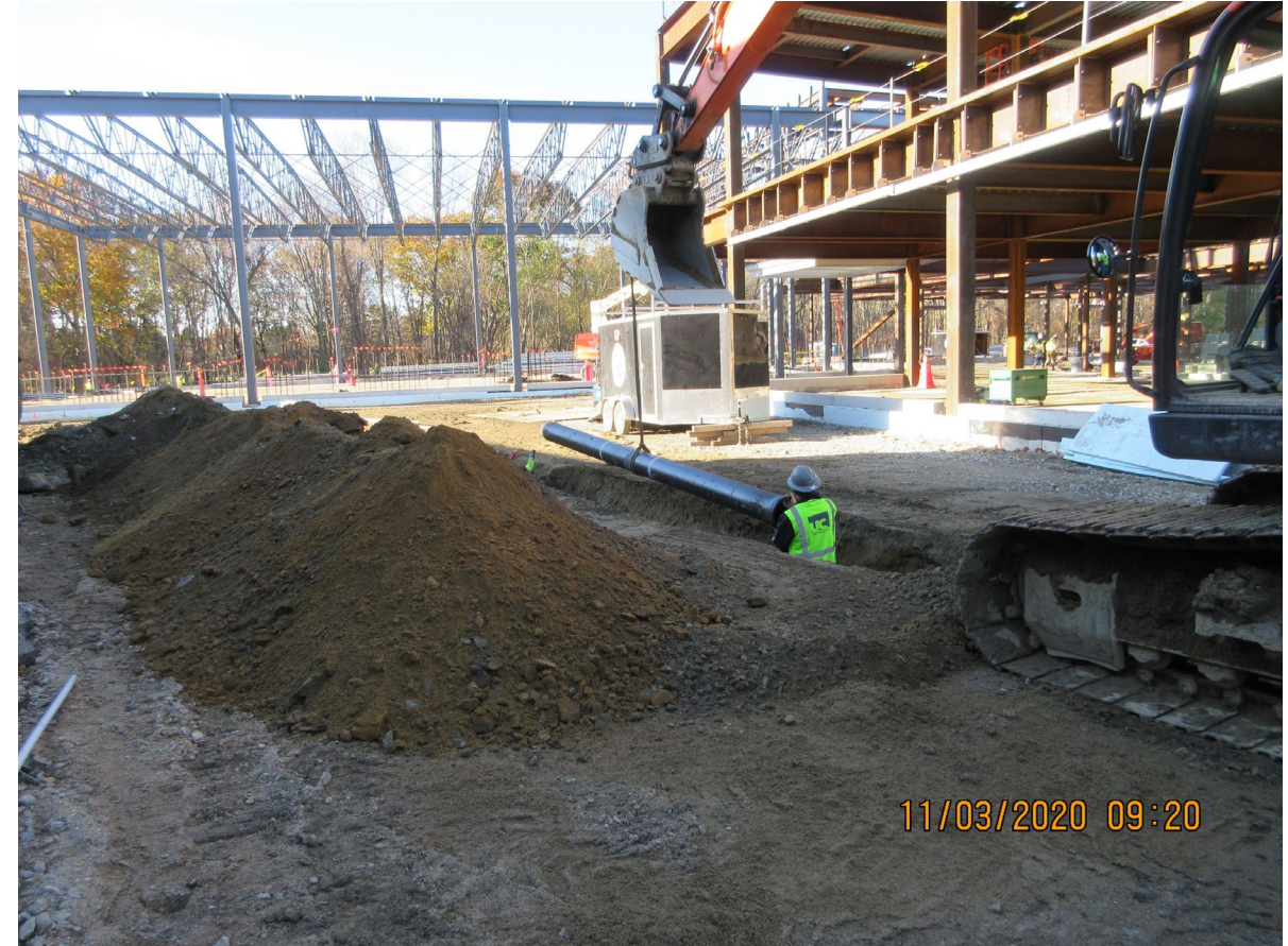
Water Line Install to Bldg. D
