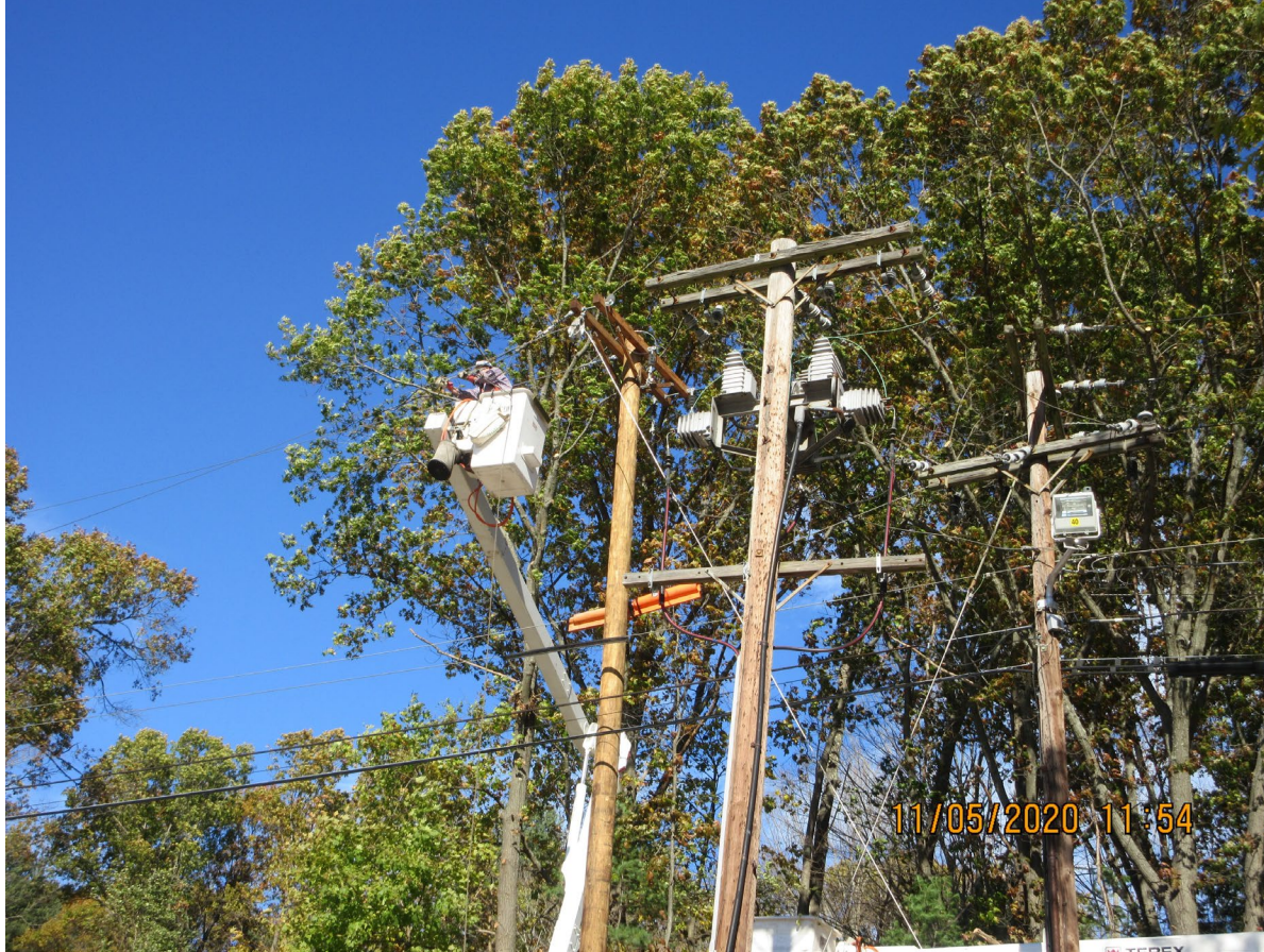
NGrid Clearing Trees and Installing Temp. Power & New Poles on Farm Lane
