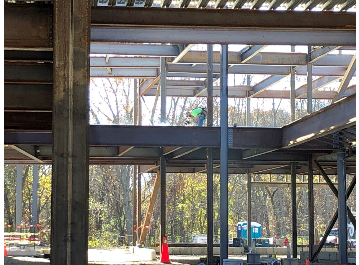
Welding Steel Decking at Building A Lobby
