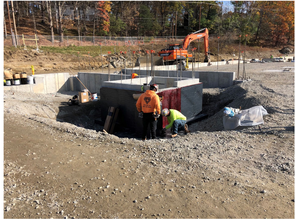
Waterproofing and Backfilling Bldg. D
